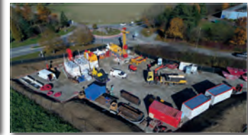
Aerial view of the GEO-01 Drilling site
