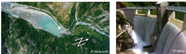
Fig. 1: Aerial view of the Sera reservoir (left) and downstream view on Sera arch dam
