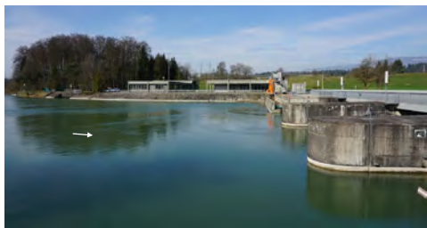
Fig. 1: Head water of block-unit HPP Bannwil with the turbine intakes in the background (Photo: VAW)
