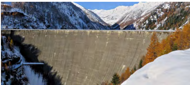
Fig. 1: Downstream view of Sambuco arch gravity dam.
