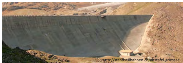
Fig. 2: Arch gravity dam Gries
