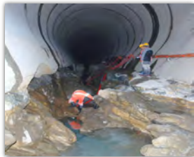
Fig 1. Hydro-abrasion at Palagnedra SBT (Photo: VAW, ETH)
