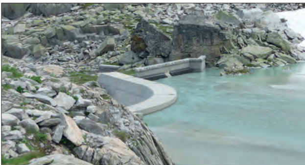
Figure 2. The Bächlibach dam which diverts the water into the Bächli gallery. The water intake is equipped with a trashrack to avoid big stones to enter the gallery. The capacity of the water intake is 7.5 m³/s.
