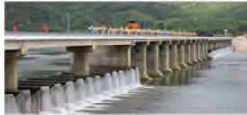
Figure 1: Van Phong Dam, Vietnam
