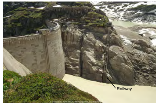
Fig 3: Lowered Grimsensee in 2006 with Spitalamm dam on the left and existing railway. (Photo: KWO)
