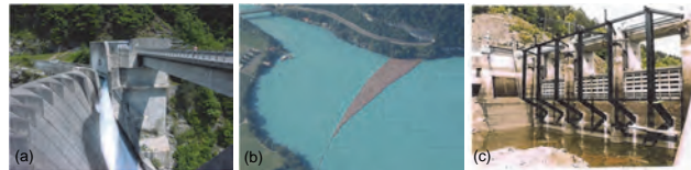
Fig 4: (a) New clear spillway with displaced weir bridge at Palagnedra Dam, Switzerland (Photo: polier.ch), (b) Floating debris barriers at Lake Brienz, Switzerland (Photo: Swiss Airforce), (c) Rack in front of spillway of Thurnberg Reservoir, Austria (Photo: bmlfuw)
