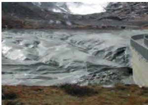
Fig. 2: Fine sediment deposits in a HPP reservoir (Reservoir Turtman, Valais; Schleiss 2005).
