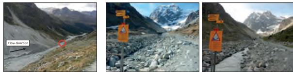
Figure 2: a) High altitude glacial catchment with water intake; b) Channel before and during a (small) purge
