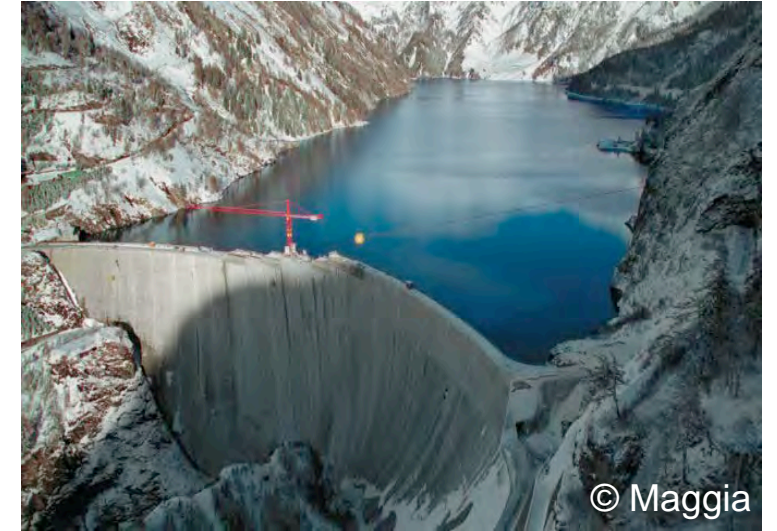
Dam heightening at Luzzzone 1998
