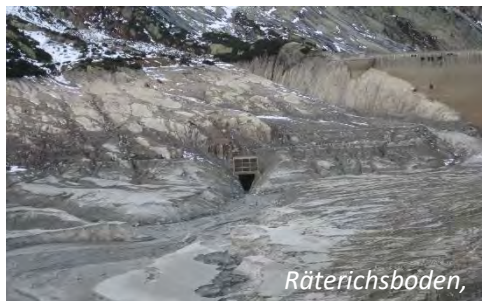
Figure 2: Reservoir sedimentation, Raeterichsboden, KWO
